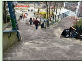
View looking west down the stairs
