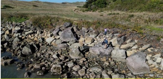
North Jetty armor: loosely interlocked boulders D_{50} \approx 1.2 \text{ m}
