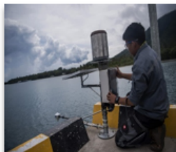
AWS – WATER LEVEL
