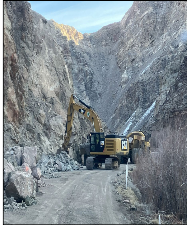
Debris Removal and Disposal
