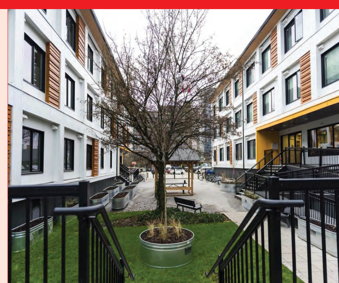
City of Vancouver Modular Housing, Cambie St., Vancouver. Source: City of Vancouver.
